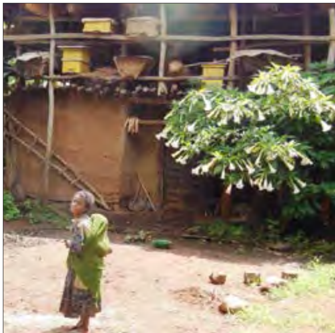
This is a typical, sturdily constructed Amhara region farm house, with eucalyptus poles plastered with mud. Its owner, a beekeeper named Gebeyehu, designed his house to accommodate his family and his bee hives. It is two stories instead of the usual one.
